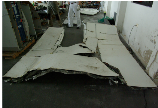
Figure 39: Ceiling of the LDMCR: with top-downwards deformation
