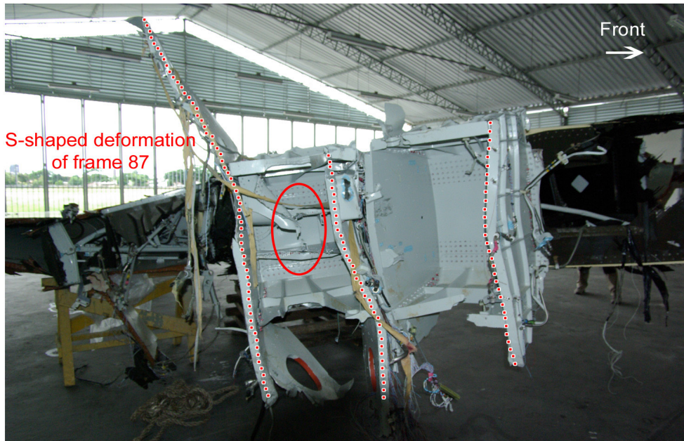
Figure 50: Frames 84 to 87: S-shaped deformation of frame 87, with frames 84 and 85 pushed in backwards; failure of the horizontal stabiliser actuator supports between frames 86 and 87 (red circle)
