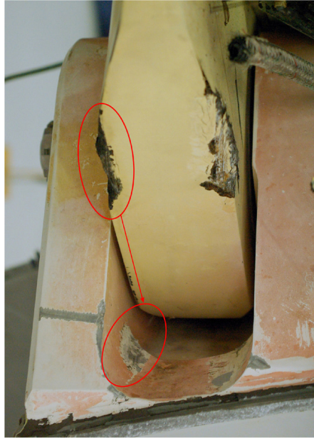
Figure 52: Rear view of the left-hand aft lug: there were marks showing a backwards pivoting of frames 86 and 87
